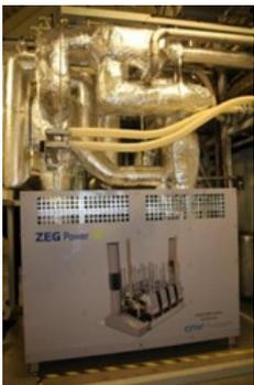
SOFC module; delivered by CMR Prototech. The SOFC-module contains 24 SOFC-stacks each made of 30 cell plates (130 x 150 mm) with metallic CFY (chromium-iron-yttrium) interconnects, delivered by Plansee/ Fraunhofer IKTS.
