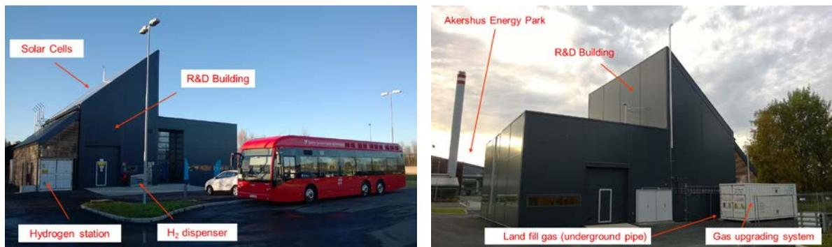
Figure 2 – Hynor Lillestrøm hydrogen station for refueling of FCEVs (left) and Test Center for RD&D (right)
